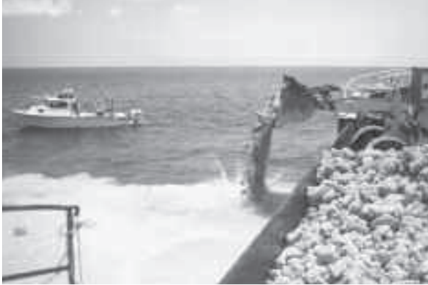
Figure D (I) Building oyster reefs with marl. (II) Building oyster reefs with empty oyster shells. (I, photograph by Ashley Harraman Burgin; II, photograph courtesy of NOAA.)
